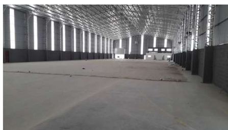
NAVE INDUSTRIAL POLO INDUSTRIAL EZEIZA, BUENOS AIRES
